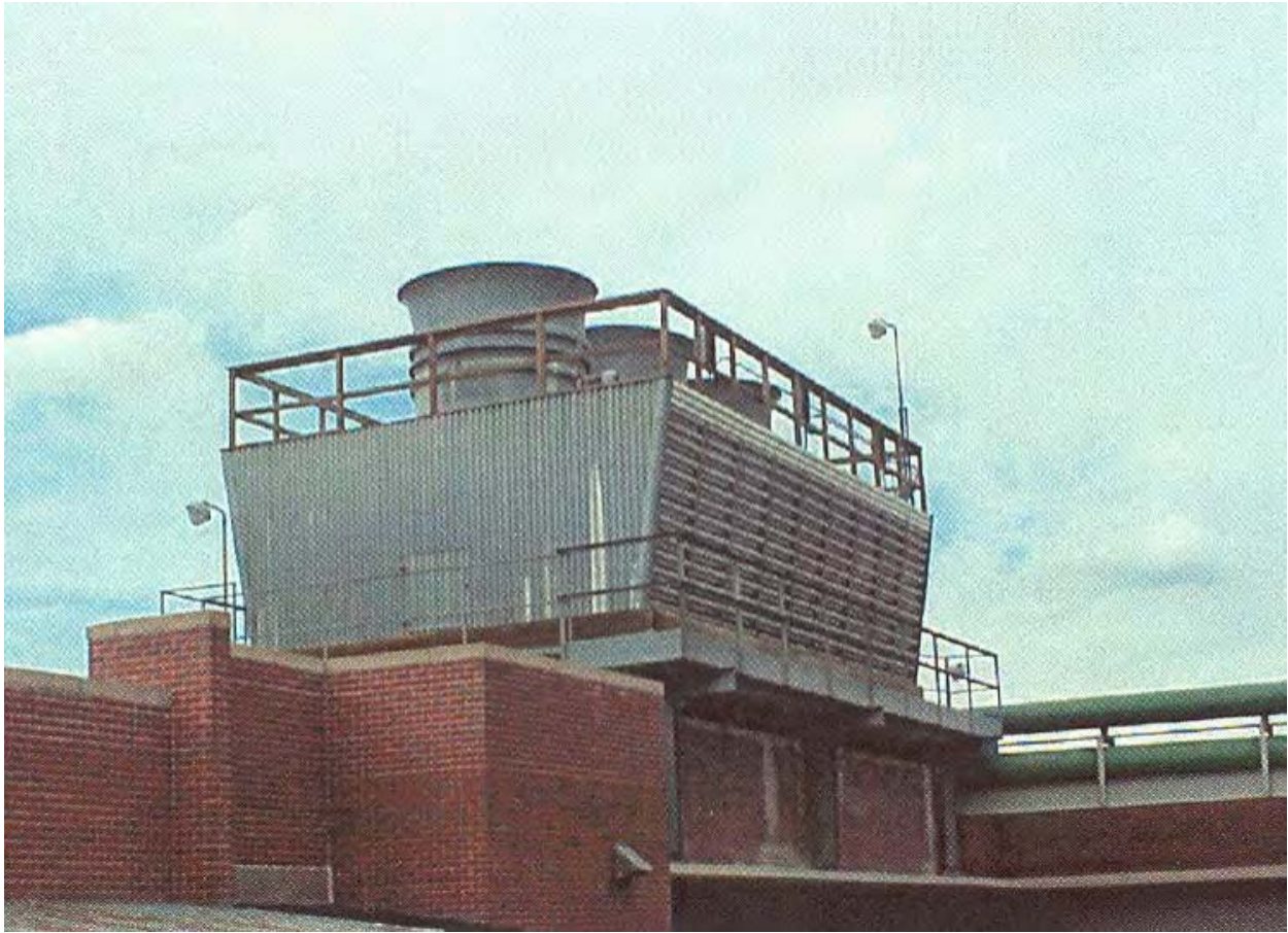
Figure 7 Cross-Flow Cooling Tower
