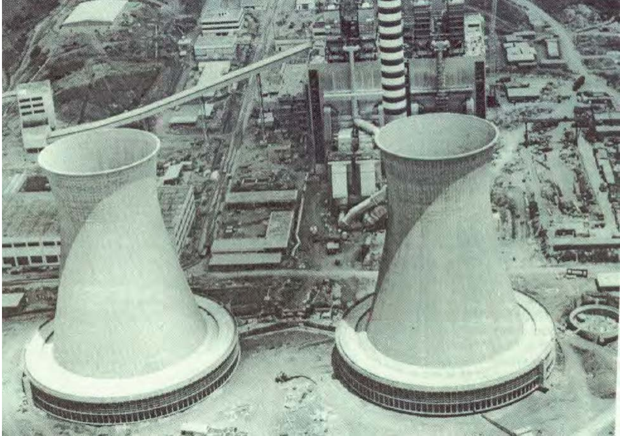
Figure 5 Hyperbolic Natural-Draft Cooling Towers
